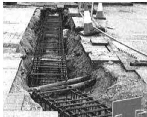
VSB foundations around underground services CPNI 2010
