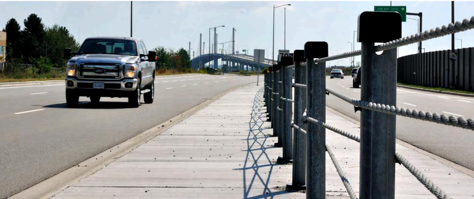
Hill & Smith are leading the way for testing as they embark on achieving a new performance rating for their Brifen wire rope VRS. Currently tested to EN1317 and NCHRP 350 the Brifen 3 or 4 rope system is recognised around the world but we are now looking to improve the specification process across global markets.
